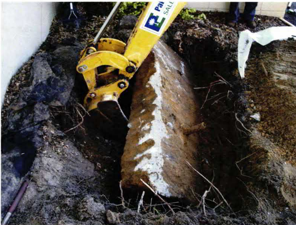
Picture 1: UST 1324Albatross excavation in progress.
